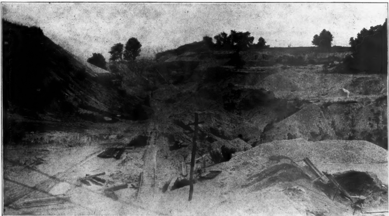
General View of Gravel Pit
